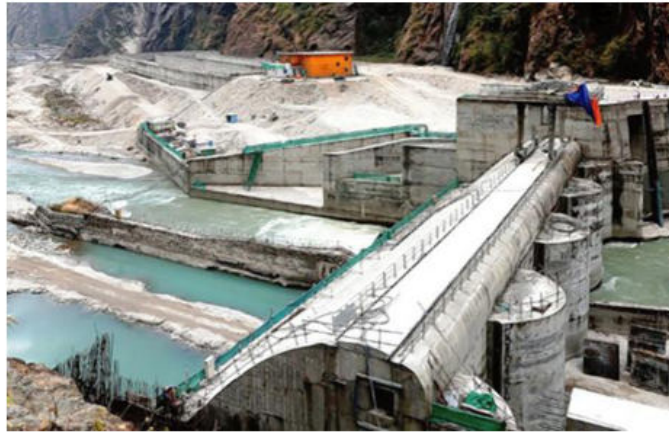
A view of the Upper Tamakoshi Hydroelectric project.
